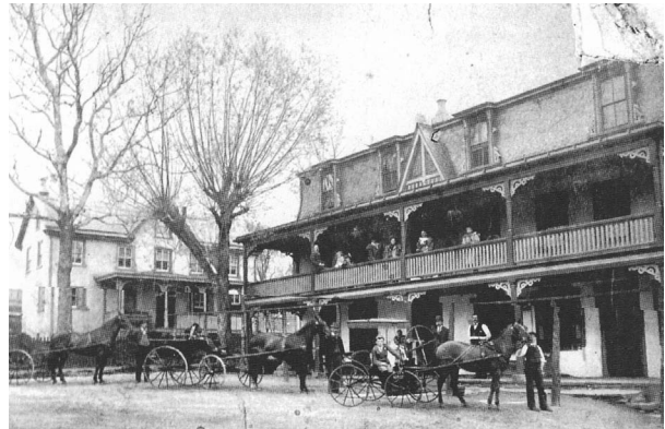
Located at 529 Bethlehem Pike, the Wheel Pump was built c. 1735 and was continuously operated as an inn until the present day. William Harmer purchased the land in 1715 from William Penn. In Colonial times, the village that surrounded the inn was called Wheel Pump, later Heydrick's Hollow, Heydrick's Dale, and finally Erdenheim.
