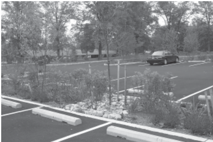
Parking lots are a natural place to trap runoff - such as here in Fischers Park.
