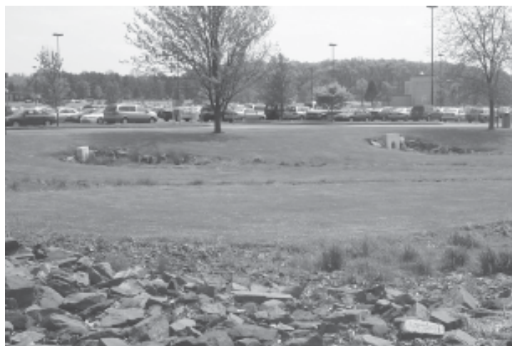
Storm drains should be maintained periodically to ensure proper functioning - clogged drains have been attributed to flood events in the past.
