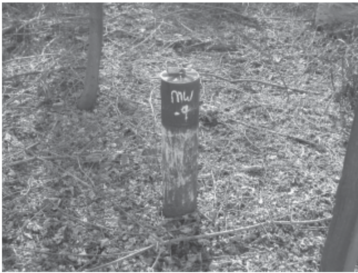
Monitoring wells are an important part of groundwater protection.
