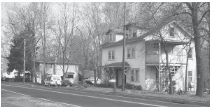
Houses within the floodplain, such as this home in Colledgeville, should be floodproofed to prevent potential future damage.
