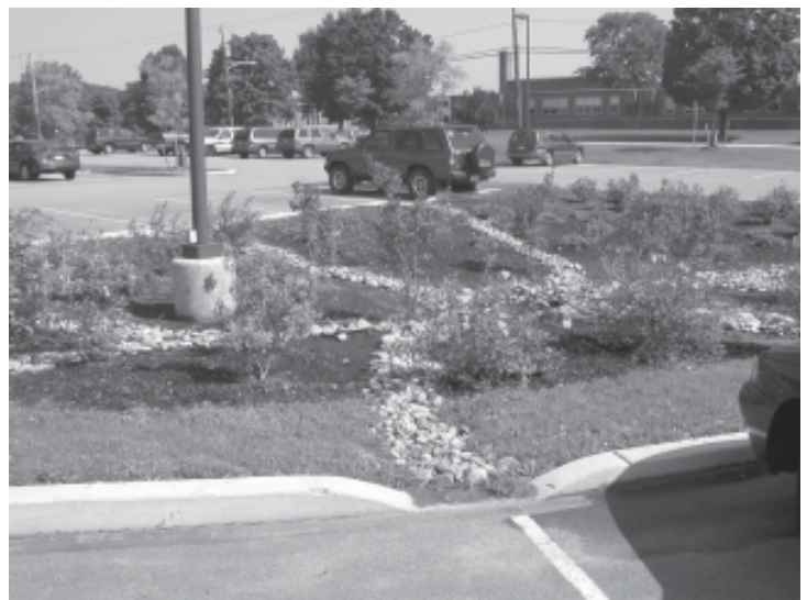
Stormwater management facilities, like this bioretention area at Upper Dublin Township's building, can improve water quality as well as provide attractive sites for plants and wildlife.
