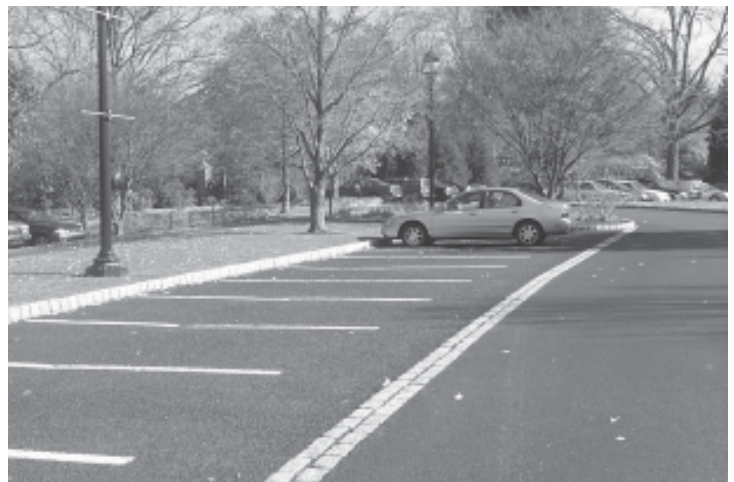
This parking lot at Morris Arboretum is paved with a porous surface that allows stormwater to soak into the ground below.
