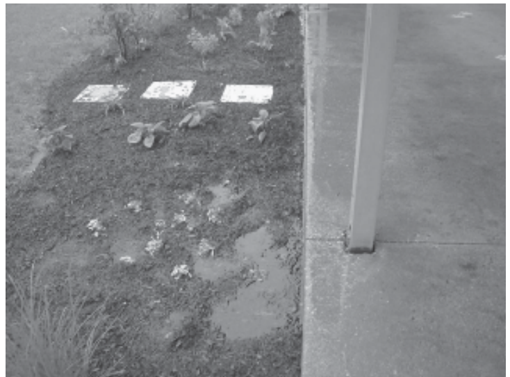
Conscientious planning of stormwater facilities, such as this rain garden, allows for environmental protection and minimized amounts of stormwater runoff.
