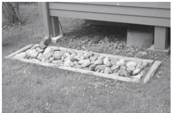
Increasing the amount of stormwater recharge, as is done with this infiltration pit, can help ensure an adequate supply of water.
