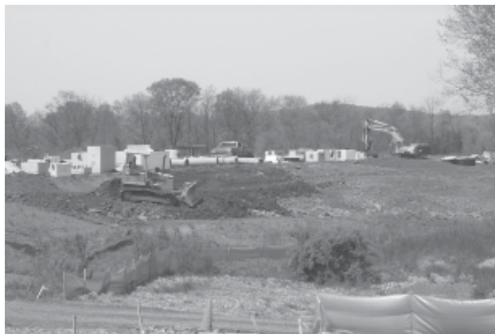
Reducing the amount of time that construction sites are cleared can cut back on soil erosion and sedimentation.
