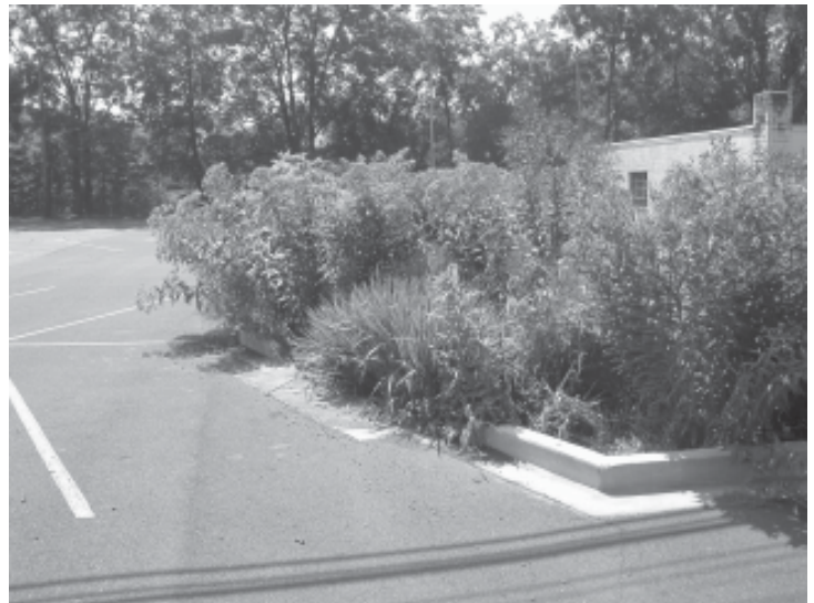
Bioretention areas use plant material to remove pollutants from runoff and allow stormwater to infiltrate back into the ground.
