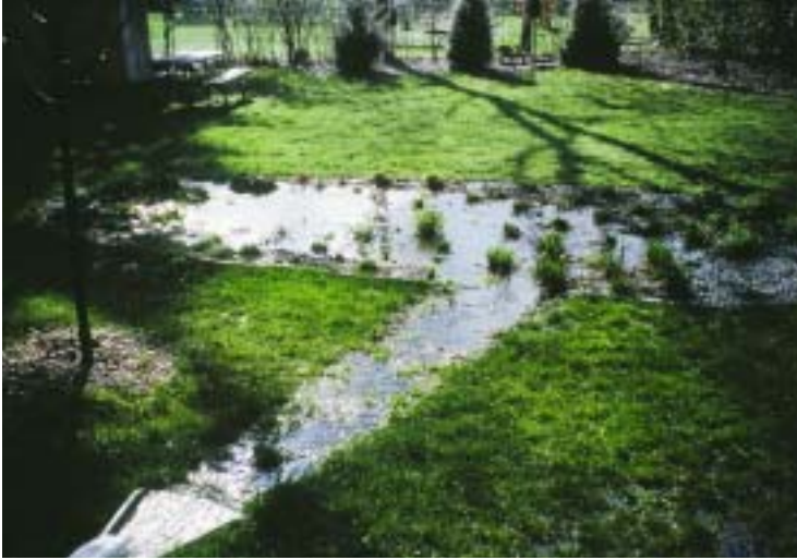
Runoff flows into a new rain garden (shown before plants are fully grown).
