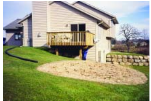
An extension of PVC pipe helps direct downspout water to this rain garden.
