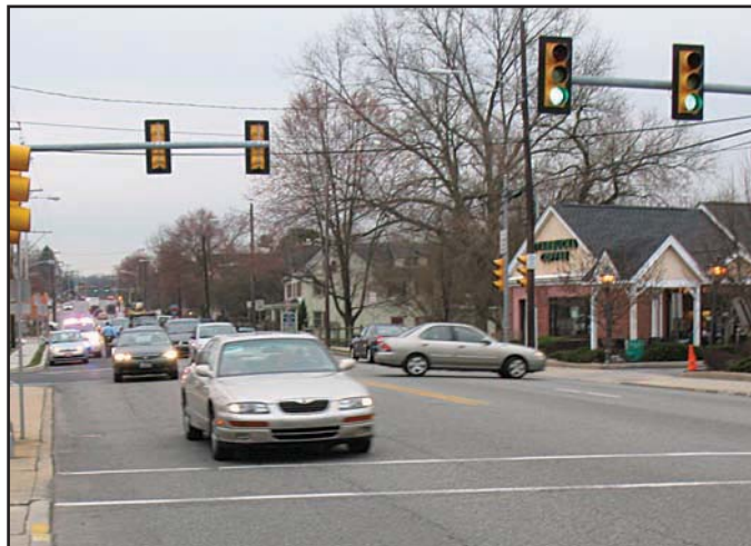
The offset intersection coupled with the Starbucks access point creates a confusing intersection with poor sight lines, and a demonstrated crash history. Source: DVRPC
