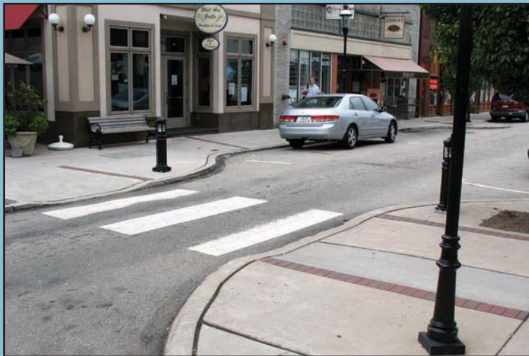
Jenkintown Borough in Montgomery County, PA installed curb bumpouts as a traffic calming measure, forcing traffic to slow down. In addition to the calming benefits, the bumpouts shorten the pedestrian crossings and create contained streetside parking. Source: DVRPC
