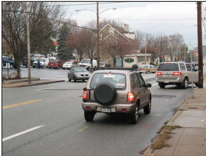
The collection of several, staggered access points by the Acme shopping center creates conflicts between turning and through traffic. Source: DVRPC
