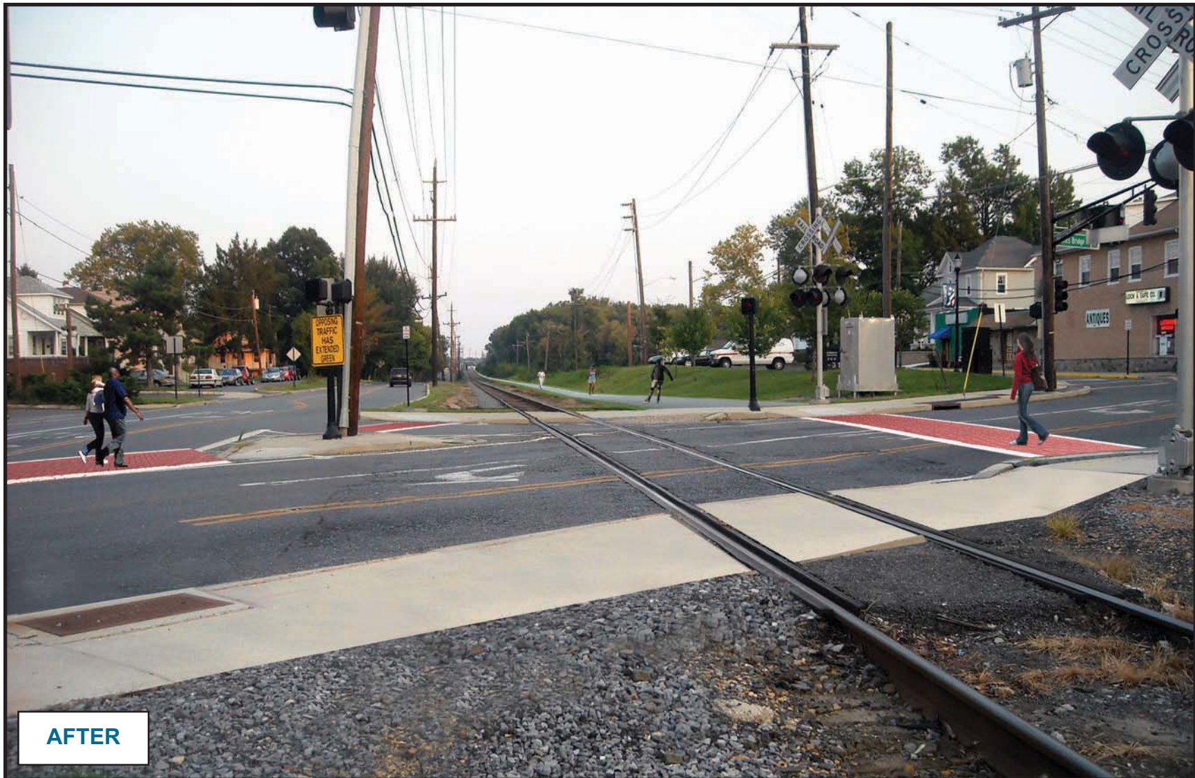
FIGURE 29: Vicinity of Clements Bridge Road, Looking East – Simulation. This image is a photo-simulation of the recommended improvements applied to the location shown on the left. Major improvements include the multi-use trail crossing over to the south-side of the railroad tracks, high-visibility crosswalks, and improved sidewalk treatments. Source: DVRPC
