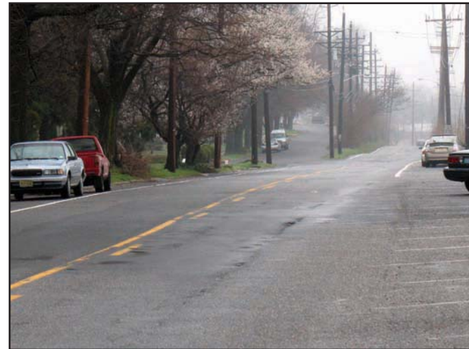
Some parts of the study area contain dashed center lines, indicating passing zones – a configuration that may not be appropriate for the corridor. Source: DVRPC
