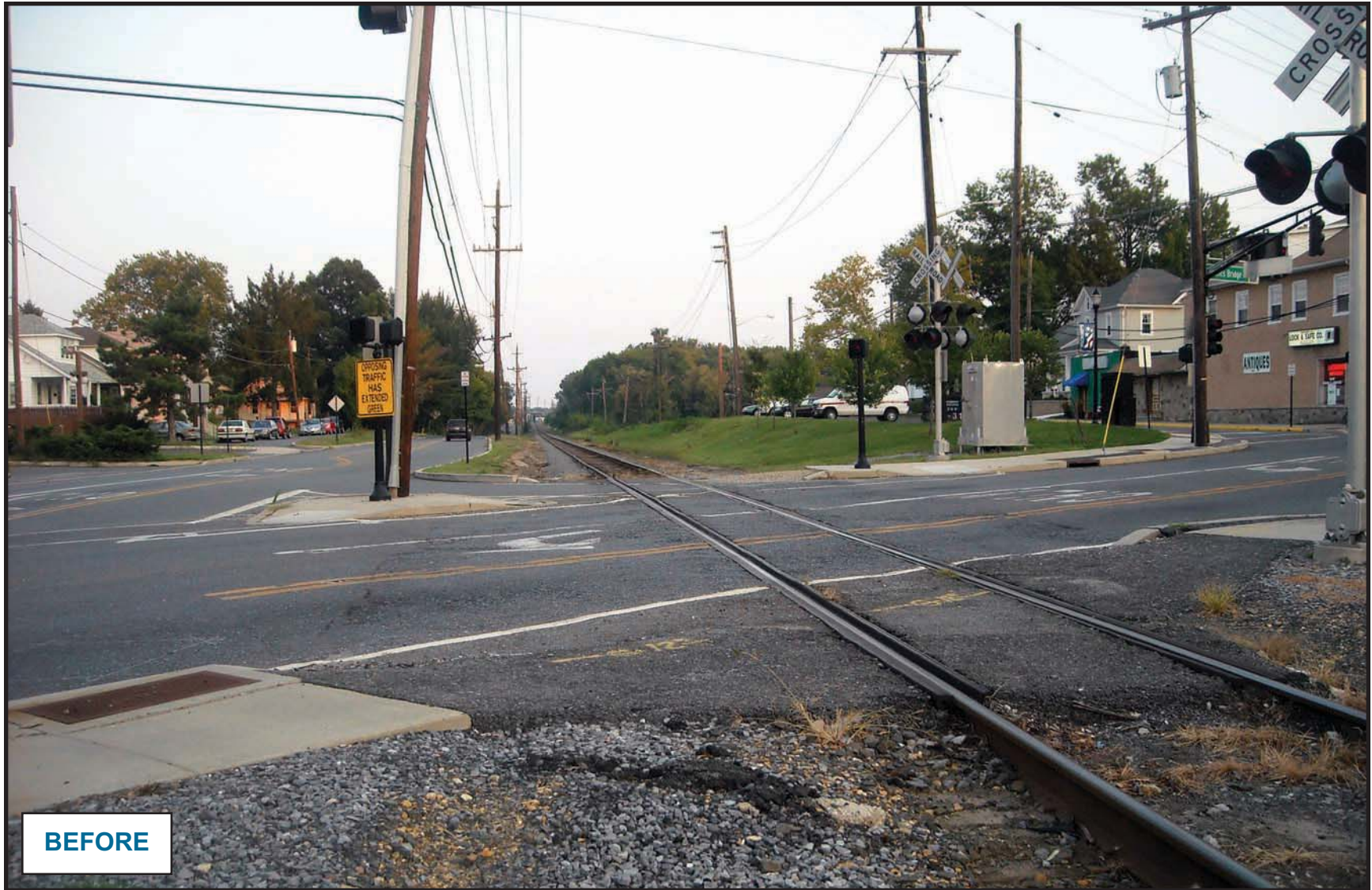
FIGURE 28: Vicinity of Clements Bridge Road, Looking East – Existing Conditions. This image is a photograph of existing conditions along East Atlantic Avenue, looking east, with Clements Bridge Road crossing over East Atlantic in the foreground. Source: DVRPC
