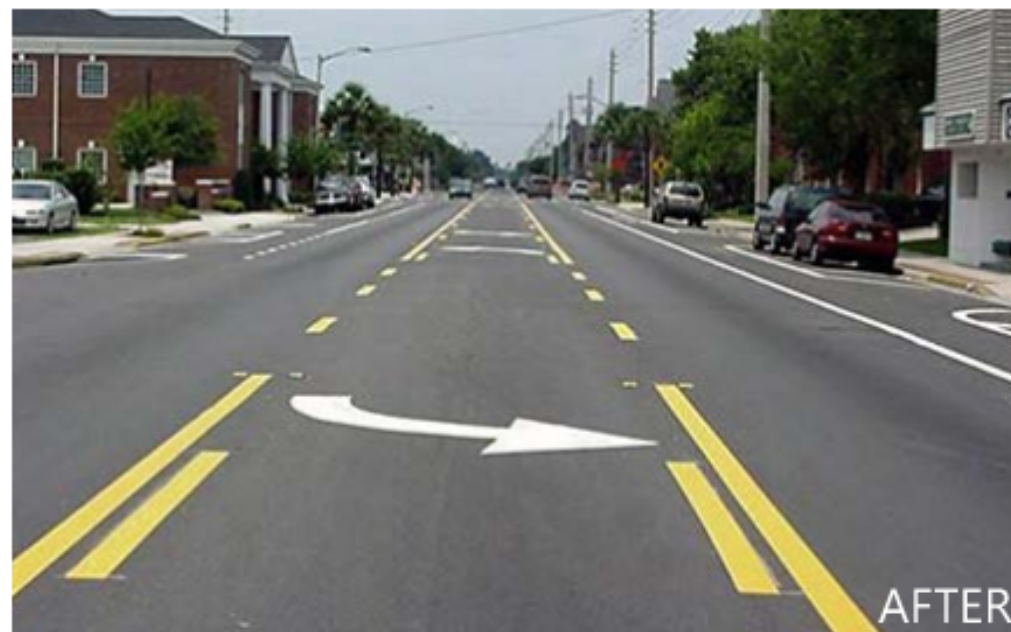
Before and after photos of a Road Diet project. FHWA-SA-17-066
