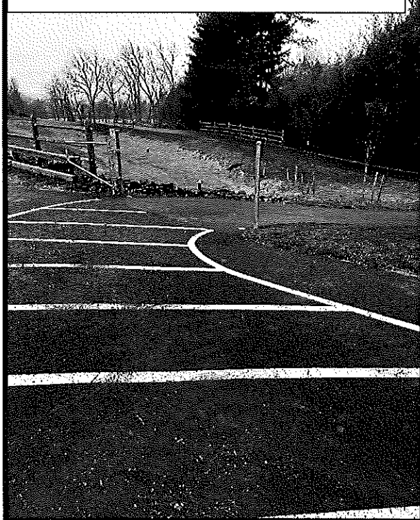
Item #18 – Emergency Access Drive – Gates
