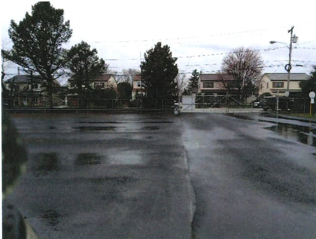
Photo 1; By: Rettew Associates, Inc., Dated: (03/24/2023)
