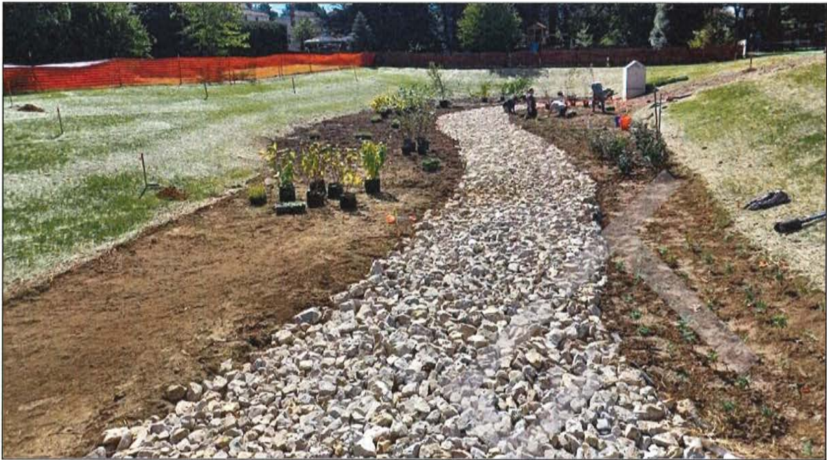
Figure 4. Integrity Avenue New Basin during construction.
