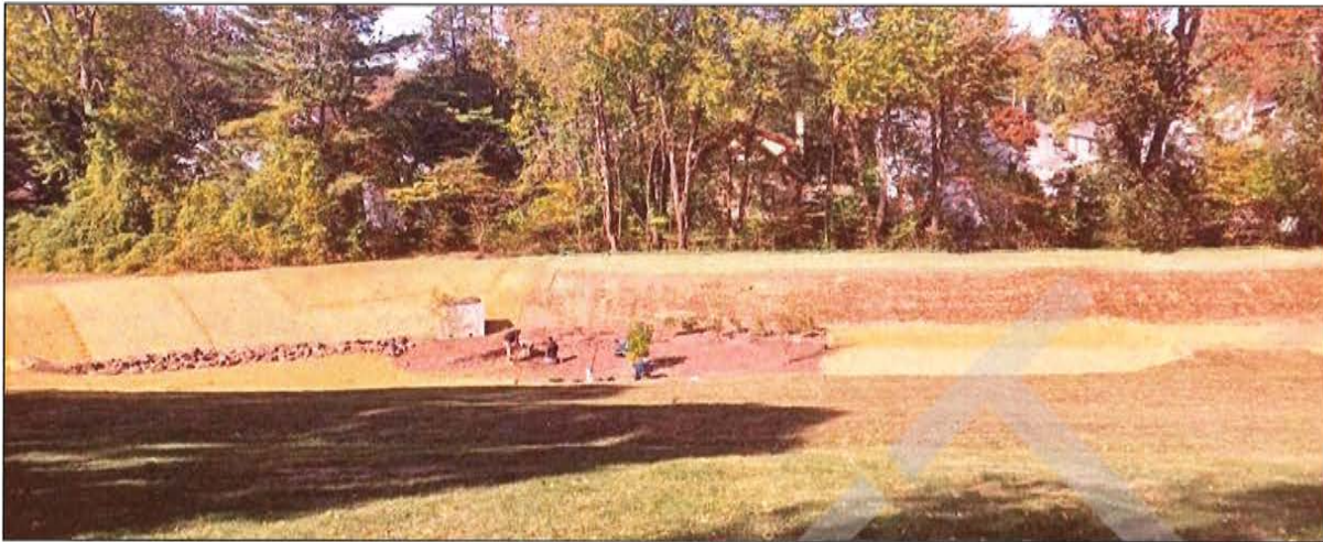
Figure 3. Skyline Drive Basin Retrofit during construction.
