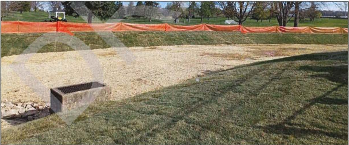
Figure 5. Sandy Run Country Club New Basin immediately post-construction.
