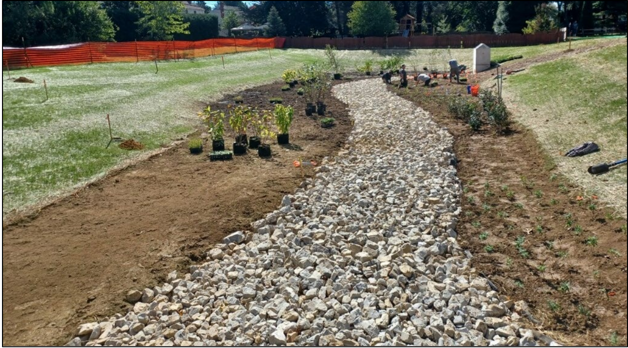
Figure 4. Integrity Avenue New Basin during construction.
