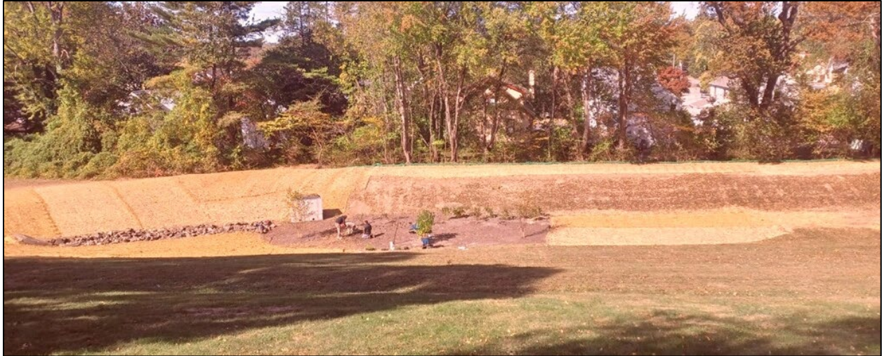
Figure 3. Skyline Drive Basin Retrofit during construction.
