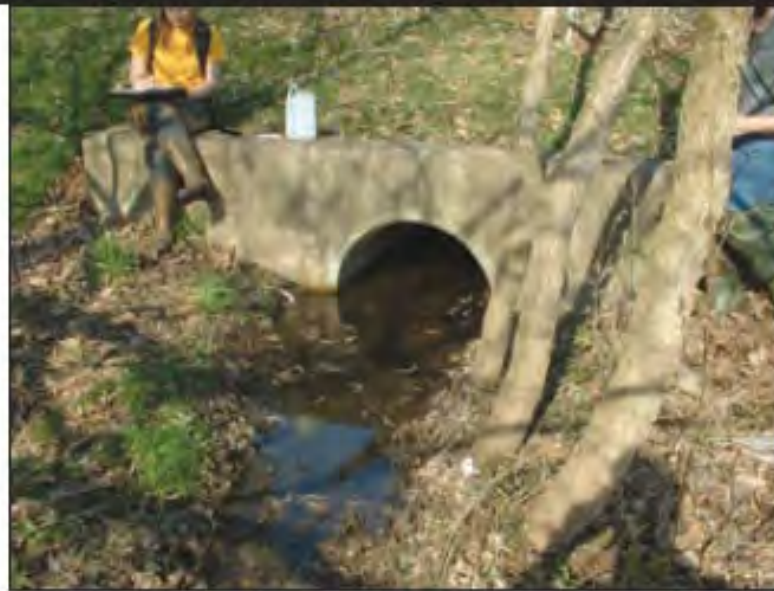
Partially submerged: Bottom is below water
