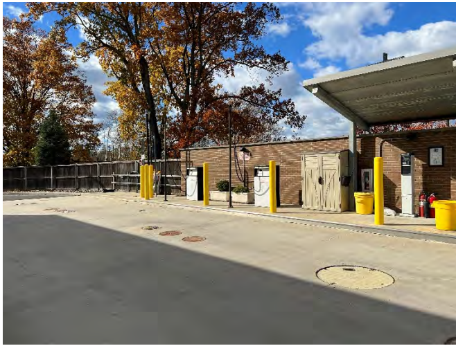
Figure 4: Township Vehicle Fueling Station
