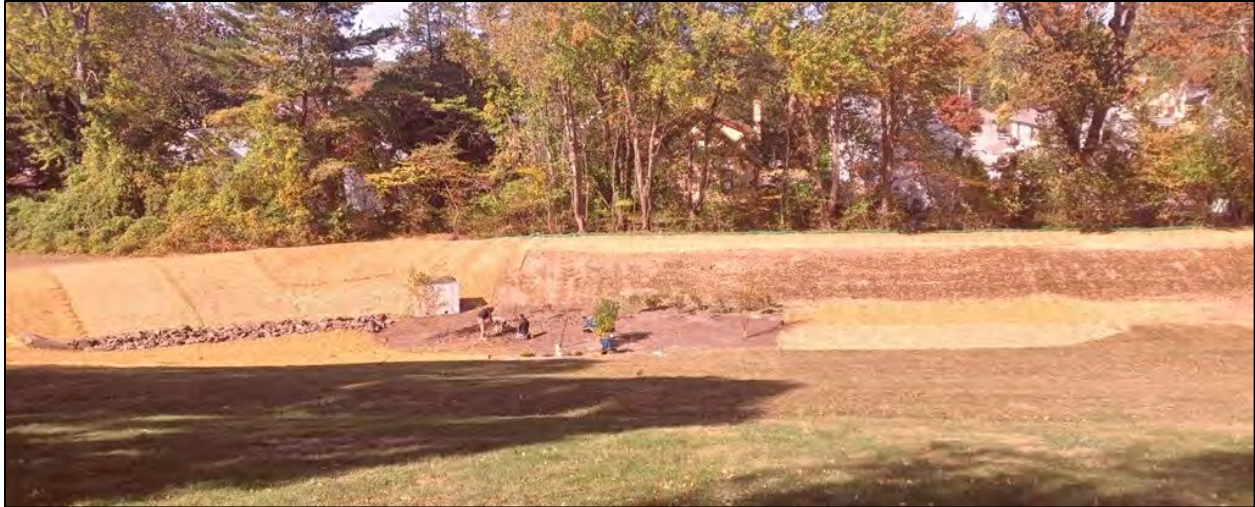
Figure 3. Skyline Drive Basin Retrofit during construction.
