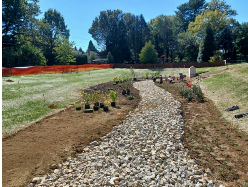
Figure 10: Construction of a stormwater basin near Integrity Avenue.
