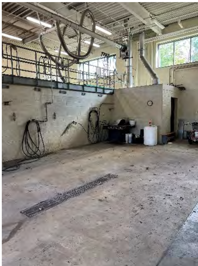
Figure 5. Designated vehicle wash bay.
