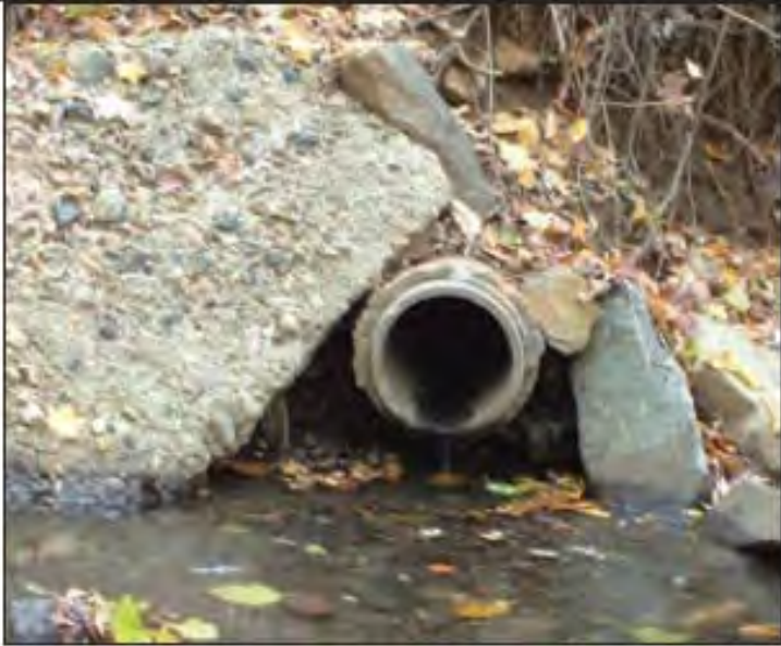
Trickle Flow: Very narrow stream of water
