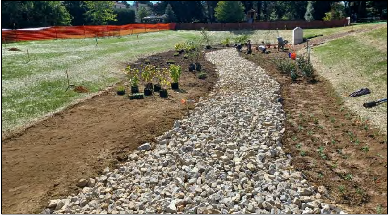
Figure 4. Integrity Avenue New Basin during construction.
