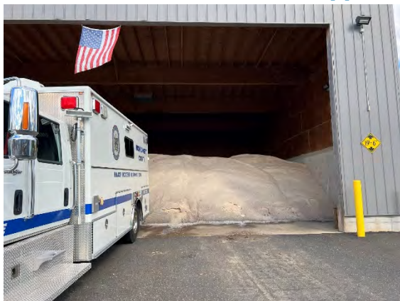
Figure 2. Salt Storage at Public Works Facility
